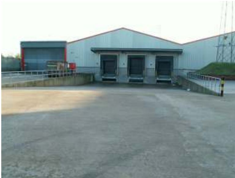
Dock levellers at Block A
